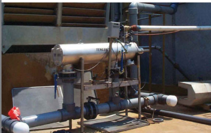
ABOVE: Tekleen's 6" model, ABW6LP-800GPM, at Bruce Foods' cooling tower. RIGHT: Tekleen's ABW3.
